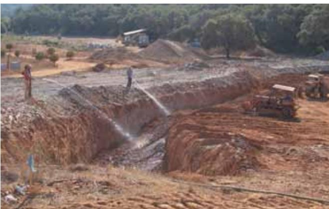
*The dam consists entirely of natural material: the sealing effect of the core is achieved by compacting earth-moist clay, loam or comparable local material.*
